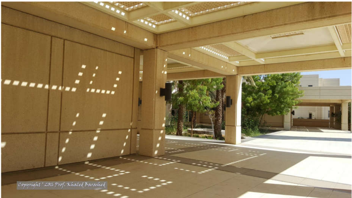
Figure 4.7, Main Entrance Court
